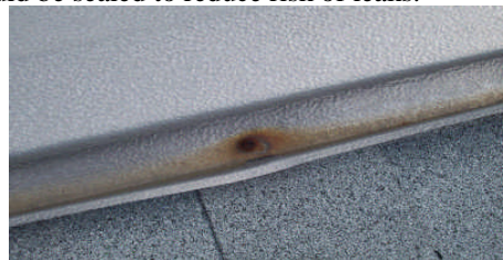
Water staining under the roof leak.
